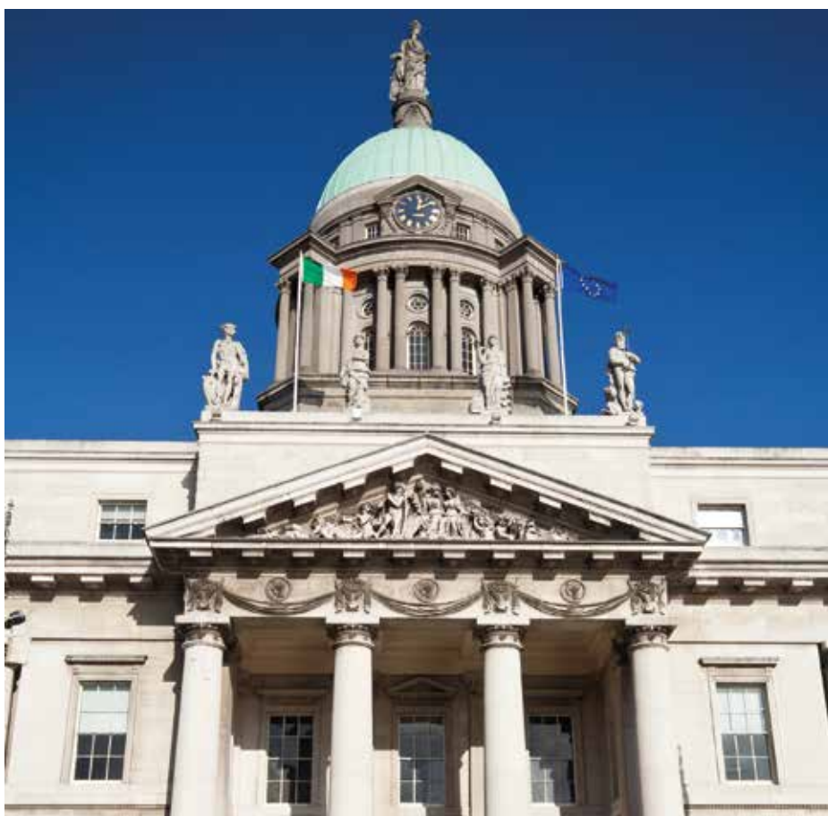
Dublino, The Custom House
